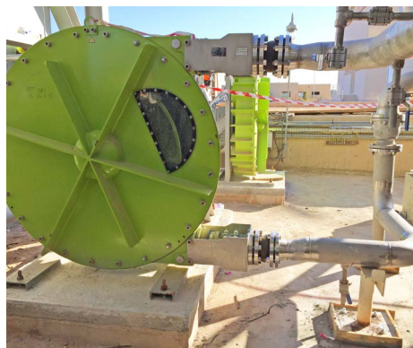
ALH125 pumping concrete
